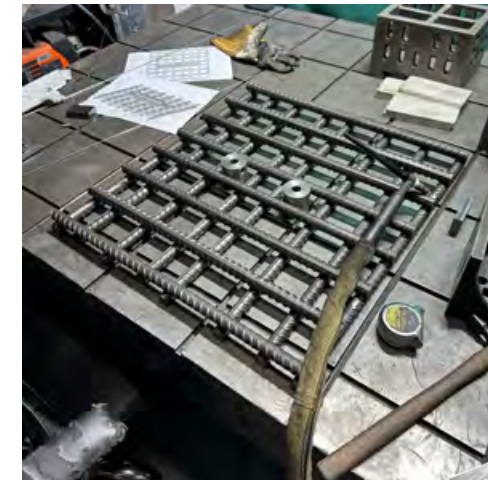
Weld Rebar Base
